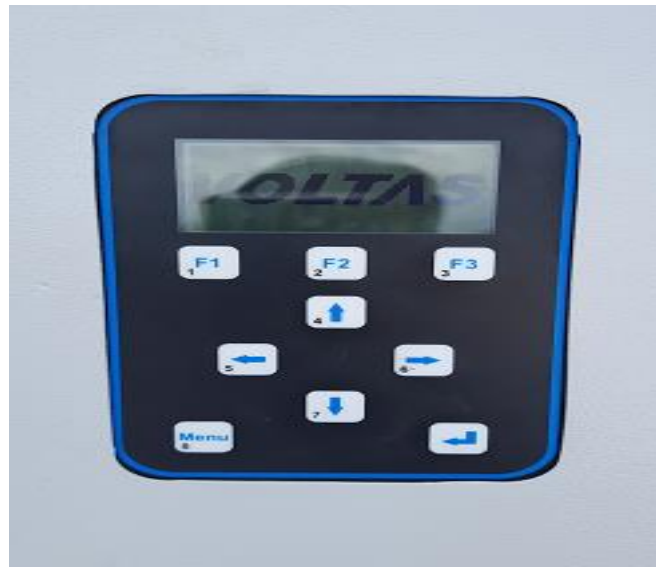
Fixing of VFD on chiller plant
