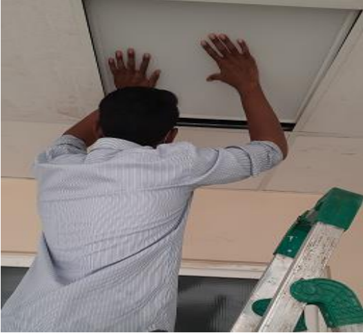
Replacement of CFL to LED Lightings
