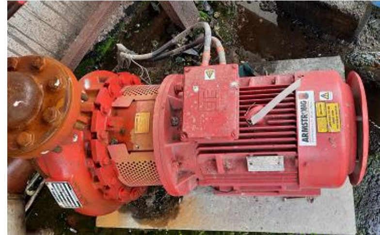
Replacement of Energy Efficient pump – chiller plant
